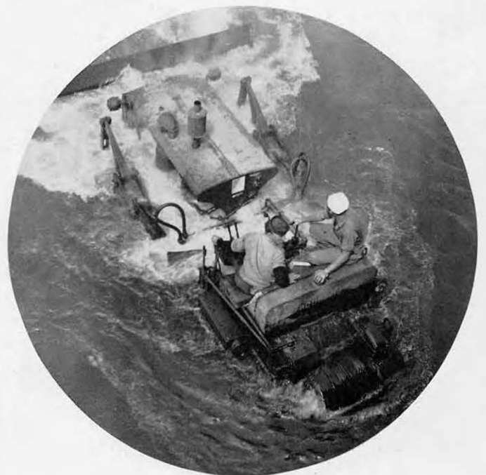
A Seabee tractor backs from shore to ramp over a submerged steel mat. The shot was taken at Port Hueneme, California.
