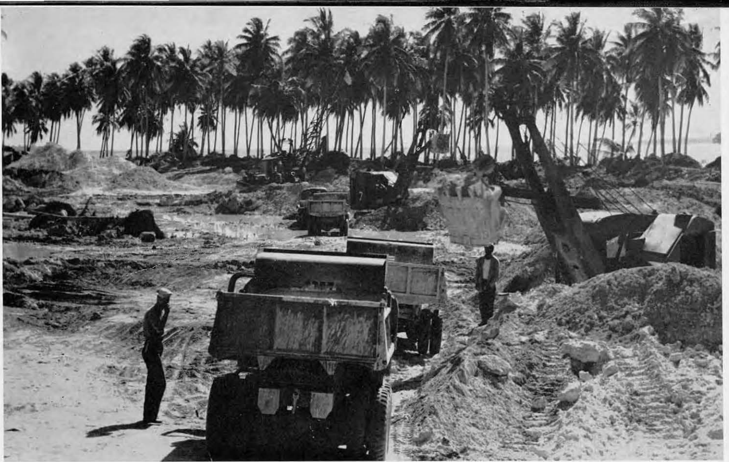
This is the Bougainville airstrip, in preparation.
