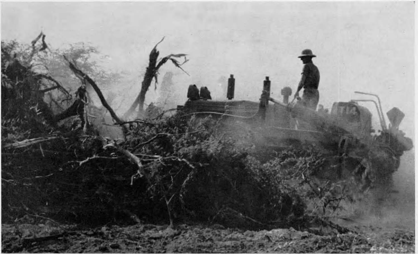
The jungle doesn't stand a chance against this Seabee equipment.
